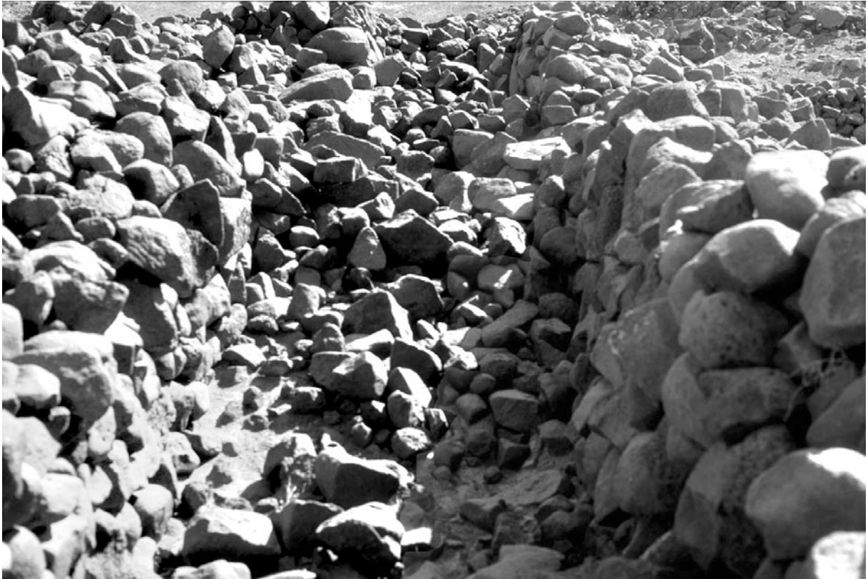
Fig. 11 The enclosed access route from the top of the island to the well shown on Fig. 10.
